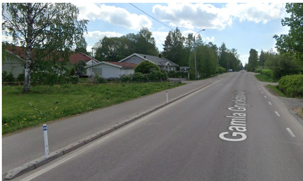
Figure 9. Image showing placement in the separator strip between the carriageway edge and the footpath and cycle path. Please note, however, that the posts on the picture are not delineator posts.
