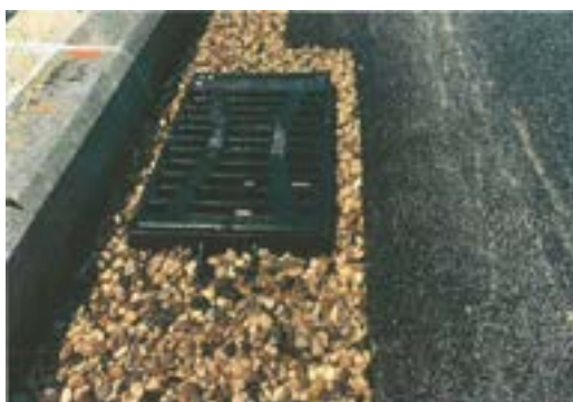
Figure 8.20: Drainage filter gutter
