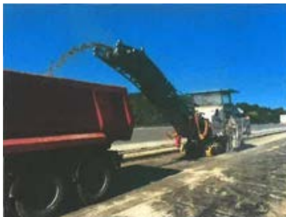
Figure 8.2: Preparation of the concrete surface c)
