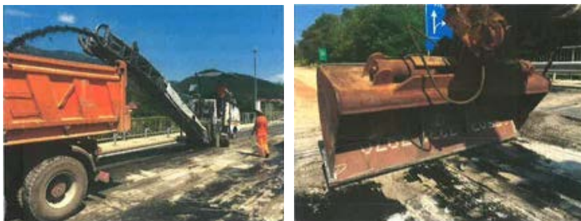
Figure 8.1: Preparation of the concrete surface a) and b)
